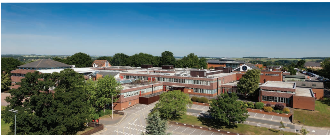
Buildings on the current school site
